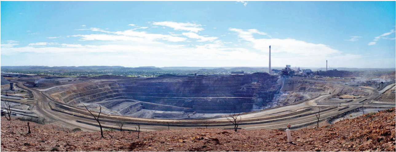
Figure 4 View of the Black Star pit – part of the Isa Mine complex.
